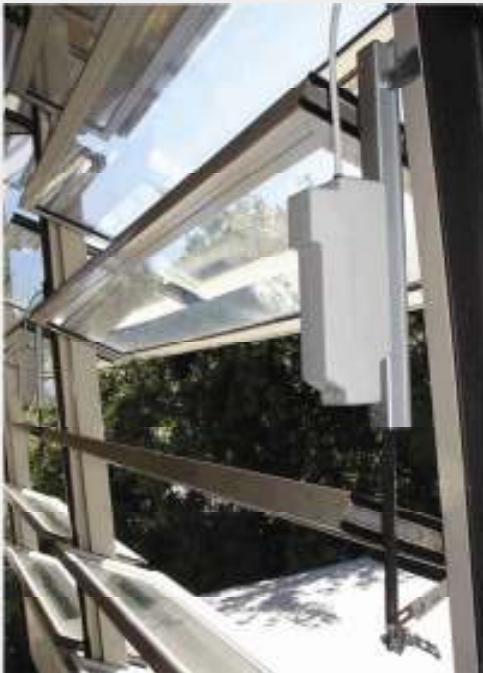
Solarhomes natural ventilation system at Bluebridge ferry terminal
